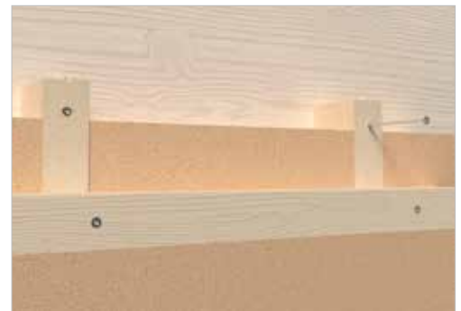
TTUFS screws in light wall framing.
