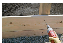
Exterior timber element fastening
