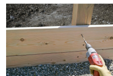
Exterior timber element fastening
