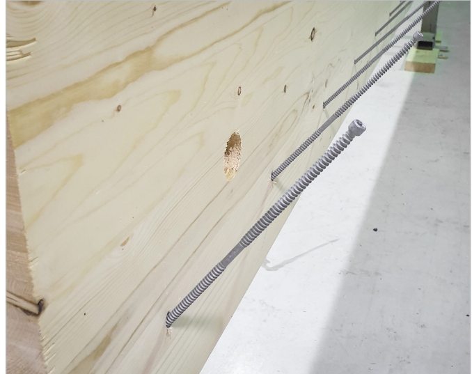
SWD screws installed into a CLT wall-to-floor.
