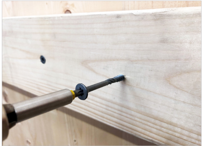
Ledger fastened with TTNFS screws.
