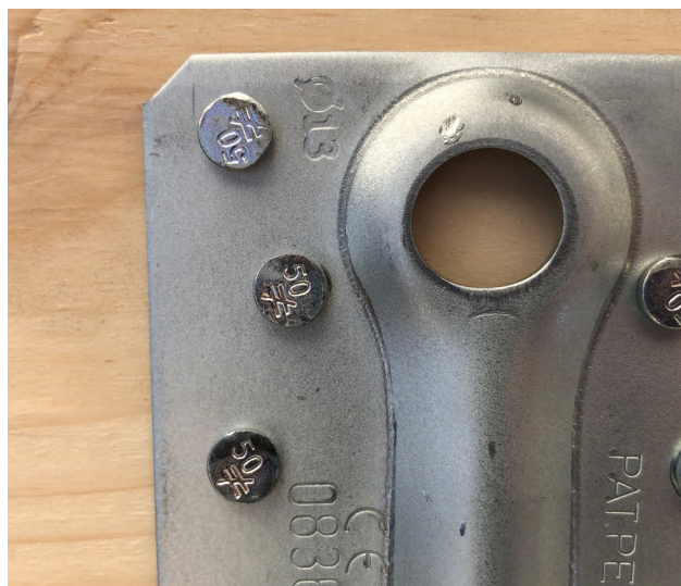
Stamps on the connectors together with the stamps on the head of the nails makes it easy to audit the installations afterwards.
