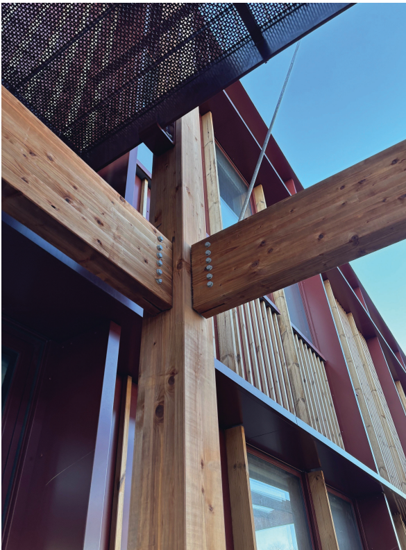
Here you can see Simpson Strong-Tie's BT4 concealed beam hangers
