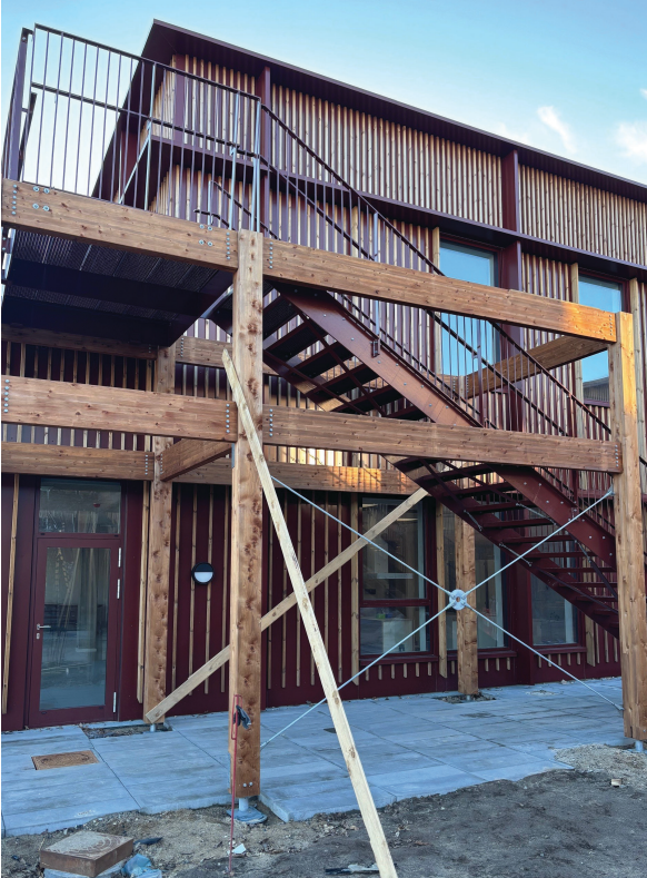
Here you can see Peikko's rod system and Simpson Strong-Tie's connectors
